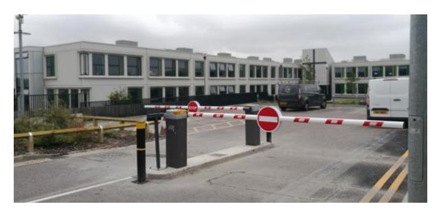
The RAPID electro-mechanical barrier is designed to regulate rapid vehicle access in intensive applications, such as at the entrance of a car park and residential areas.
